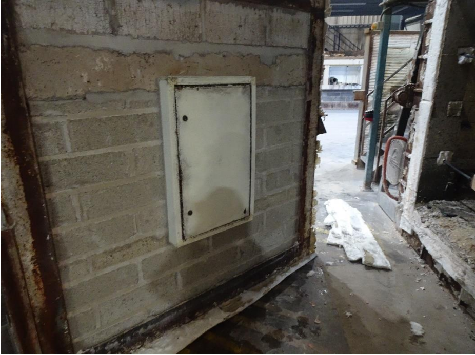
The exposed face of the electrical box shortly after the test
