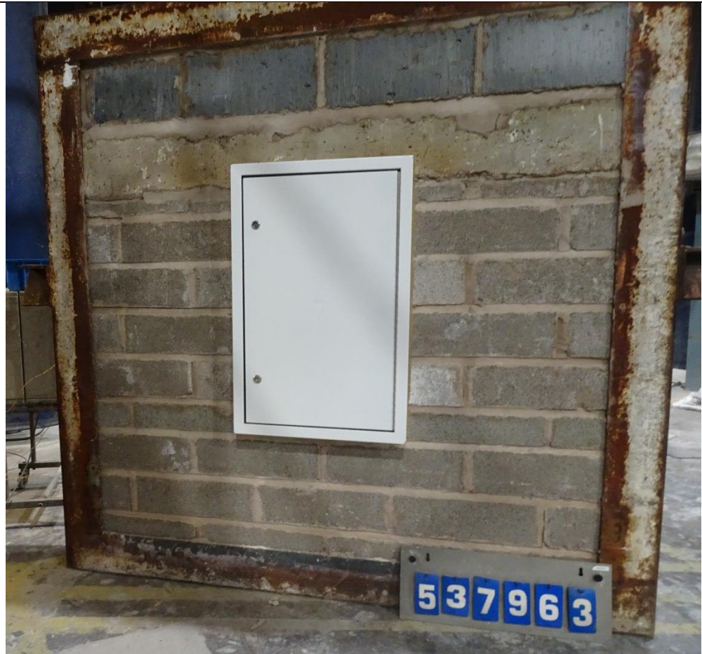
The exposed face of the electrical box prior to the start of the test
